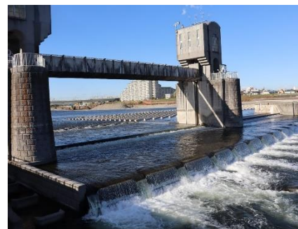
用水への取水口 宿川原の堰
